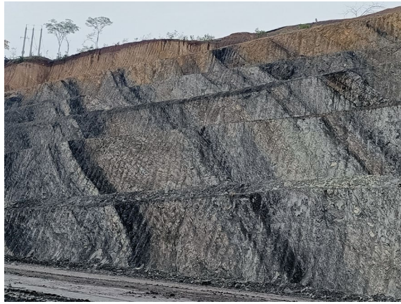
B. J_n = 2 . One joint set – bedding in a coal mine (note: slope is 60m high), very low RQD, Colombia.
