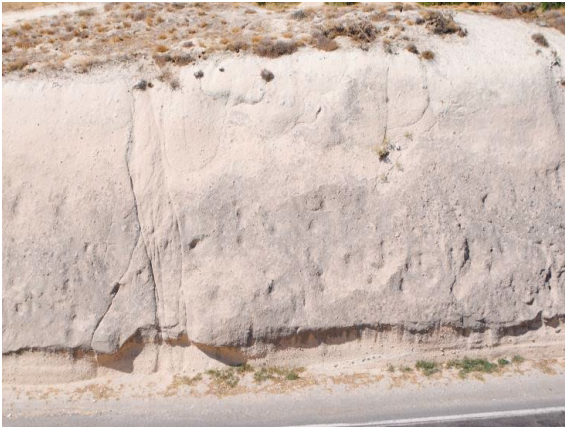
A. J_n = 1 . Occasional random joints in road cutting in tuff (note: slope is 8m high), Türkiye.
